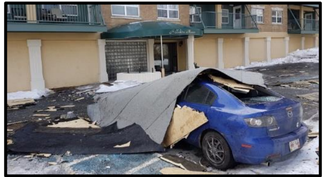
Wind Damage to an owner's vehicle at Hillshire Manor Condo Corp. - 2017
